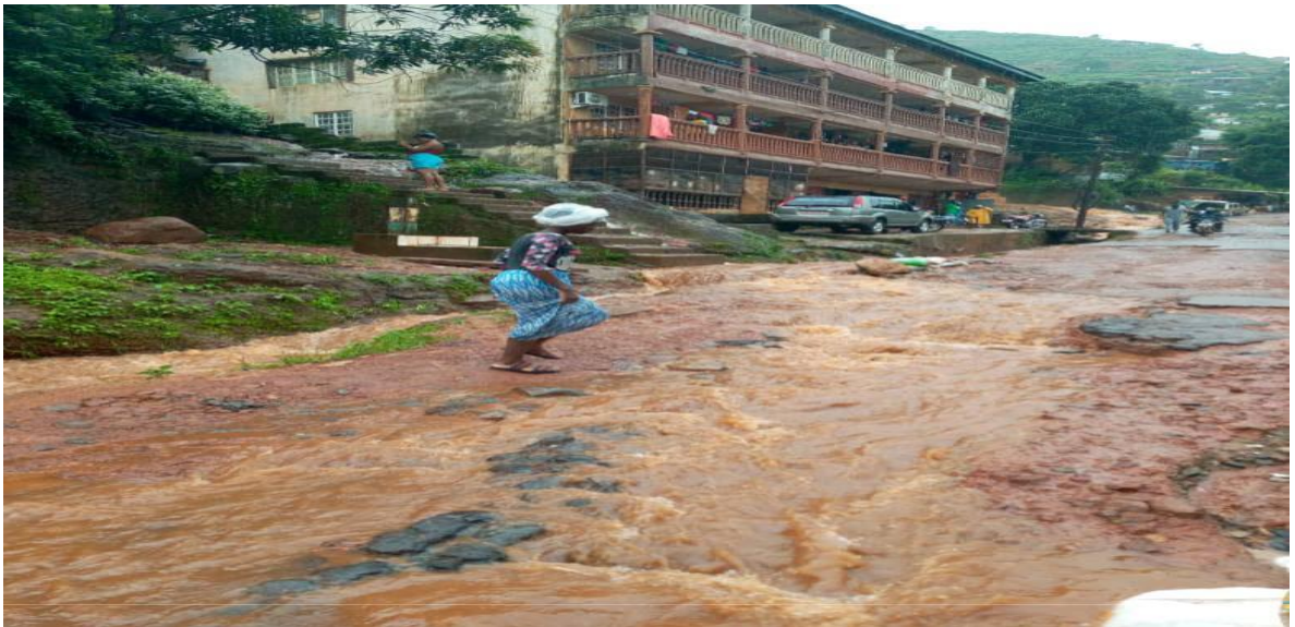
Figure 5: Improper drainage system (Source: field data collected by author, June 21, 2019)
